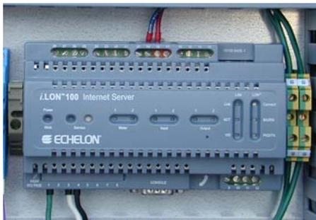
*Pictured: Internet Server to provide internet communications either through DSL or dial up connection*
