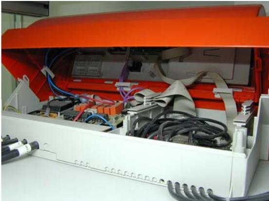
Picture showing open rear end of Dekamatik B style boiler control.
